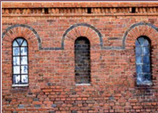
Stary mur Alte Mauer
